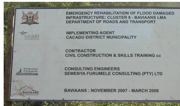
Figure 5:2 Rehabilitation project of flood damage infrastructure in Baviaanskloof.
