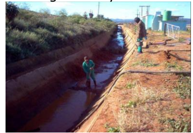
Figure 4:11 Periodically canal cleaning.
